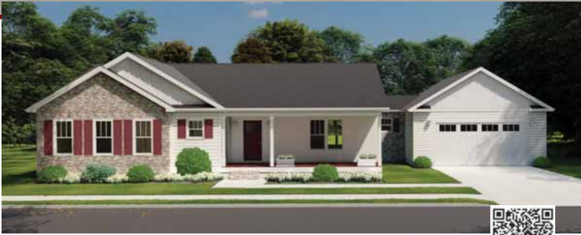
Shown with site built garage.
